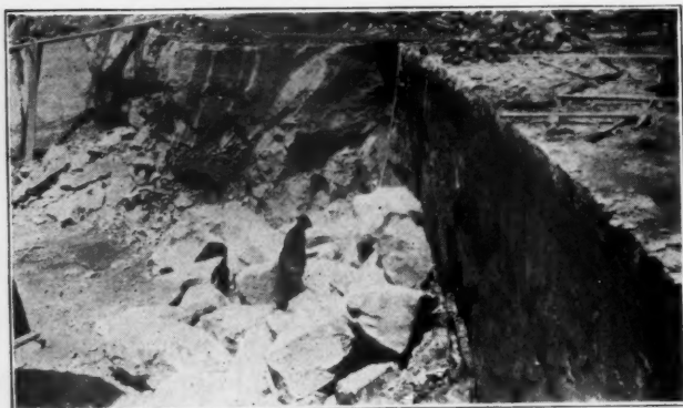
Drilling Boulders with Air Drills
